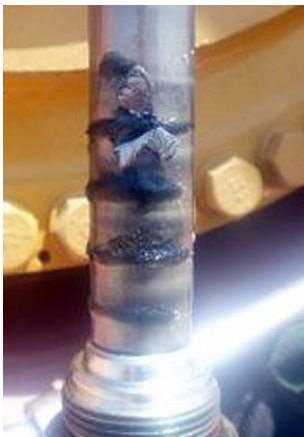
Magnetic plug showing sludge buildup
